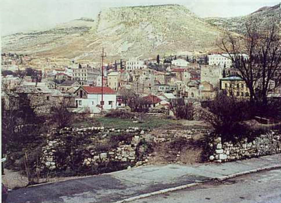
The site before reconstruction
