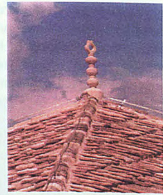
Mosque: a roof detail
