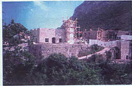
Mosque during construction
