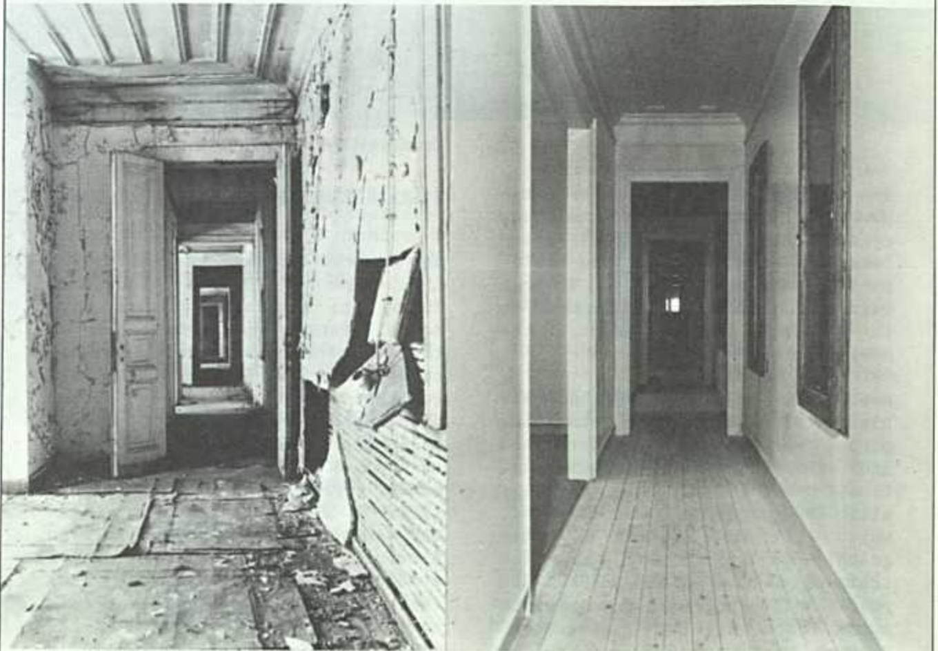
Interior of the building before and after restoration
