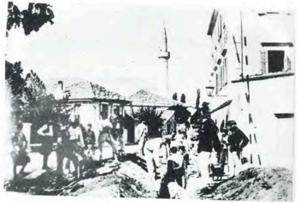
Water supply system construction at Mehdan, 1885
