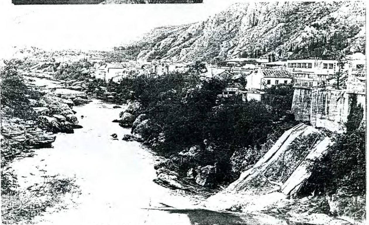
A destroyed bridge, May 1992
