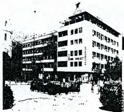
B. Administration building (1960)
