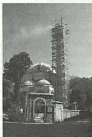
Karadgozbeq Mosque, under reconstruction
