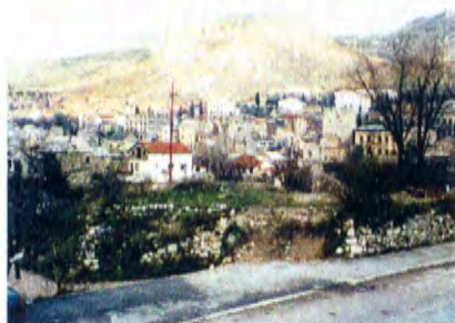
Site before reconstruction, Spring 1998
