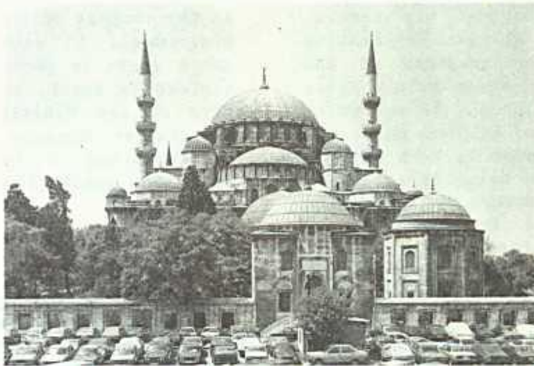
Süleymaniye Mosque in Istanbul, built between 1550-56
